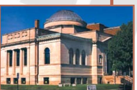
Winona Free Public Library 151 W. Fifth St. Built: 1899 NR: 1977 LH: 2001 Architects: Warren Powers Laird, Edgar V. Seeler Winona lumberman William H. Laird funded the handsome Neo-Classical library. His nephew, dean of the University of Pennsylvania architecture school in Philadelphia, was one of the architects.
