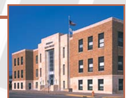
Winona City Hall 207 Lafayette St. Built: 1939 NR: 1999 LH: 2000 Architect: Boyum, Schubert & Sorenson Designed by a Winona architectural firm in the Classical Moderne style, the city hall was financed by the New Deal's Public Works Administration (PWA).
