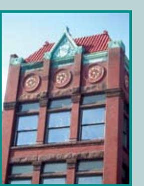
J.A. Merigold and Co. Dry Goods 59 W. Third St. Built: ca. 1868 NR: 1998 Stone rosettes and a stamped copper cornice ornament this three-story brick building.
